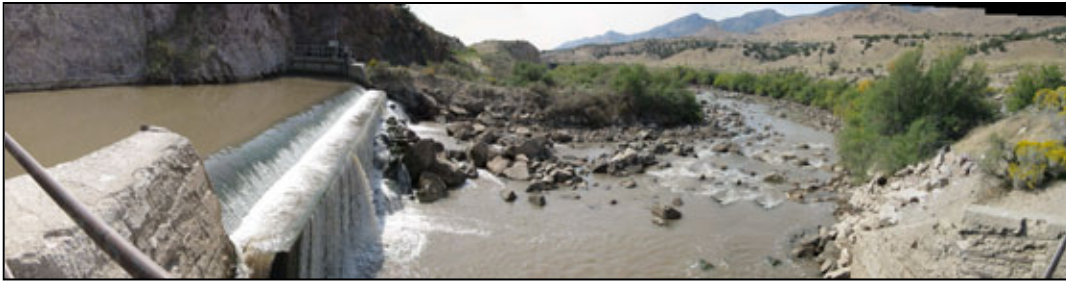
Photo 5. Turbid water at the Central Canal Diversion during September 2012.
