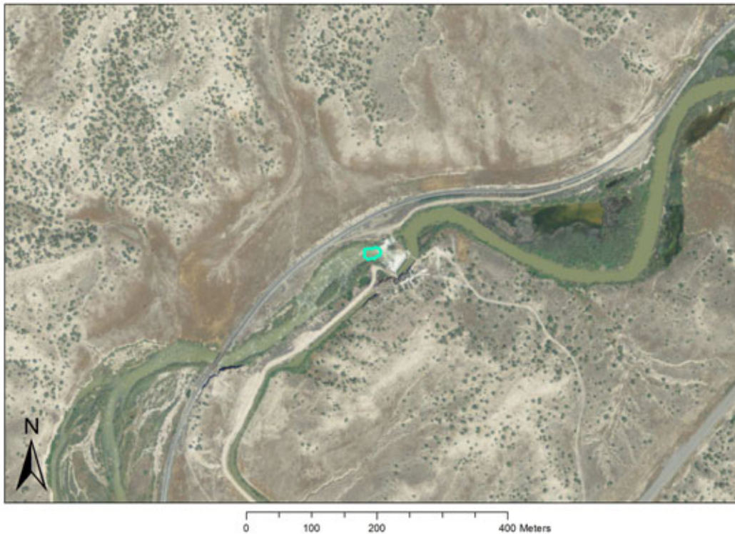
Aerial Photo A8. Central Canal Diversion location (blue polygon).
